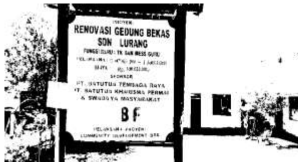
FIGURE 2 RENOVATION OF THE FORMER ELEMENTARY SCHOOL BUILDING IN LURANG VILLAGE
