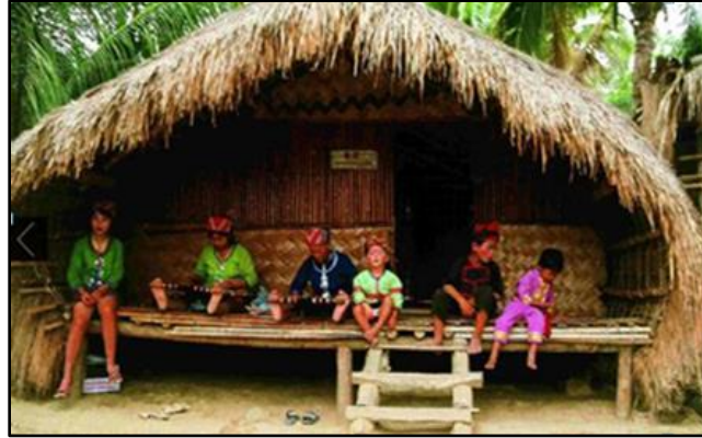
FIGURE 1 ELEVATED BOAT HOUSE IN THE INITIAL STAGE
