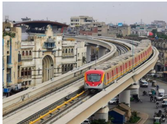
FIGURE 7 ORANGE LINE METRO TRAIN SYSTEM (OLMTS)
